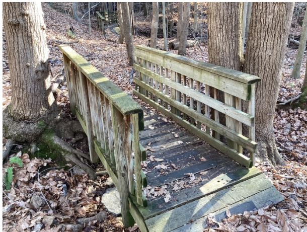
Shorter bridge overview
