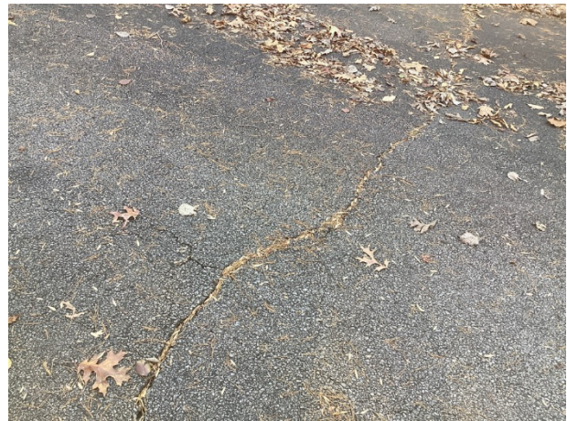
Pavement cracks
