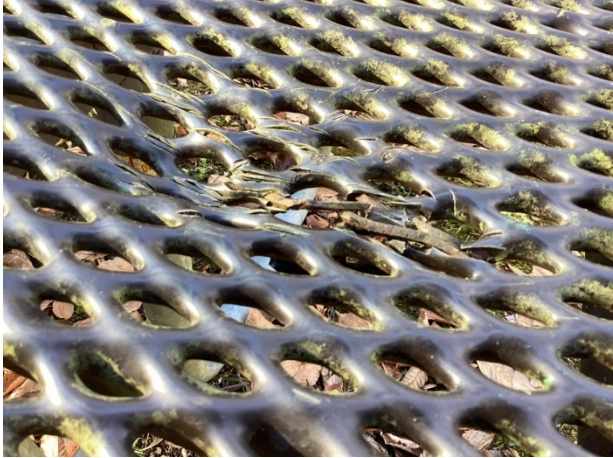
Picnic tables damage
