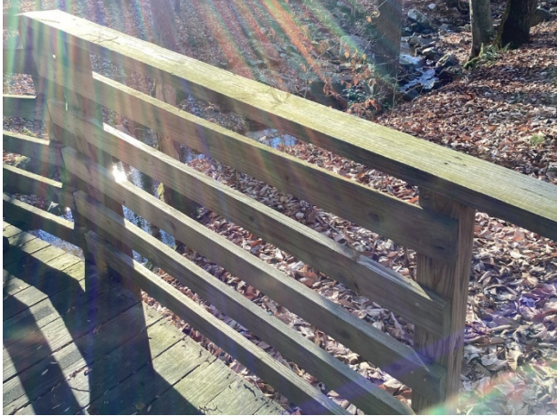
Longer bridge repaired section
