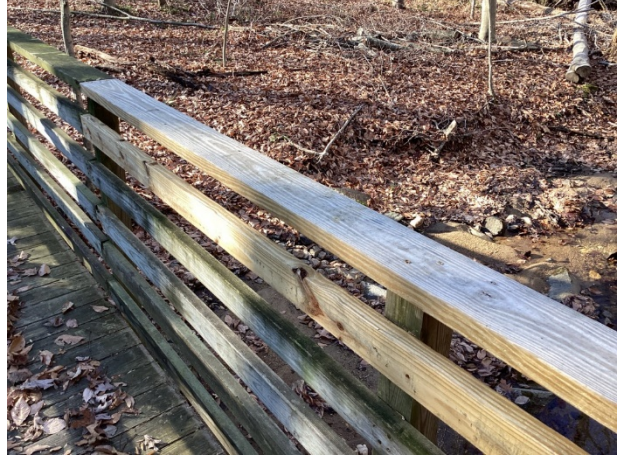
Longer bridge repairs
