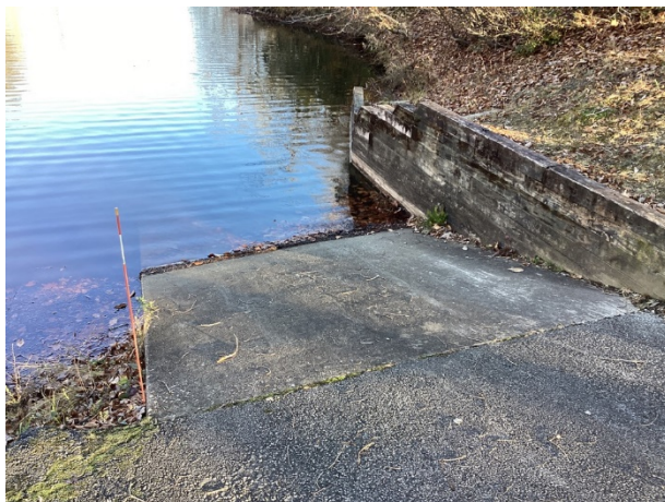
Concrete boat ramp overview
