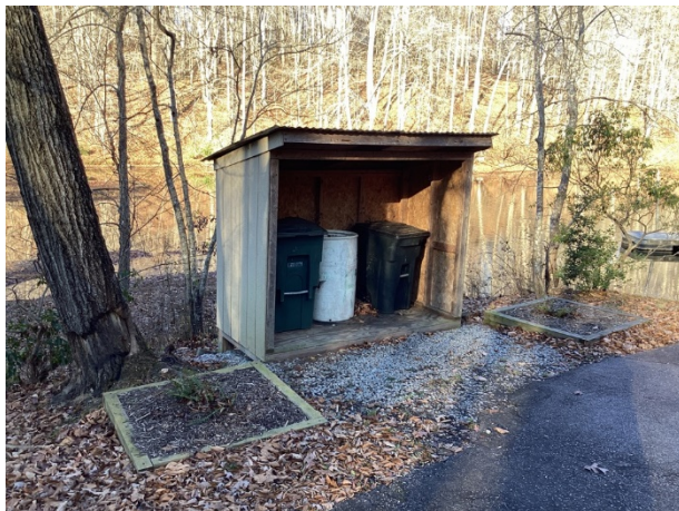
Trash shelter overview
