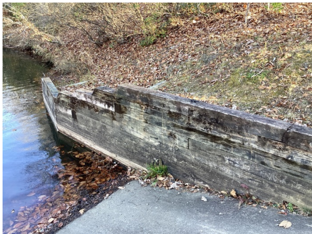
Timber retaining wall overview
