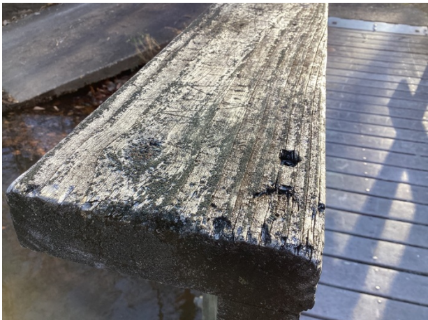
Wood deterioration
