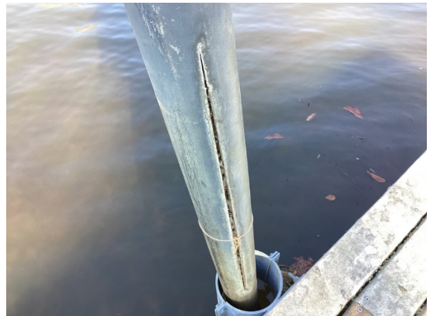
Pile damage
