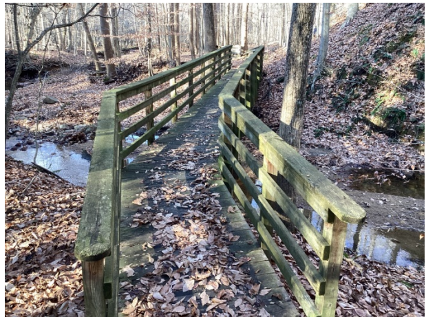
Longer bridge overview
