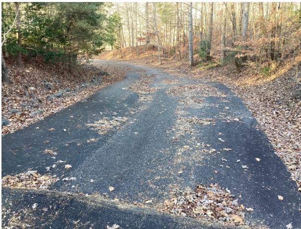
Asphalt pavement street overview
