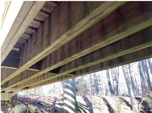
Longer bridge underside profile
